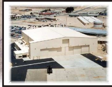
Corrosion Control Facility, Edwards Air Force Base; G and W Builders, Inc., builder.
