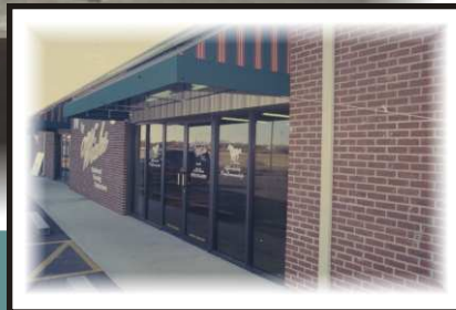
Firebaugh Complex; Sargent Construction Co. builder.
